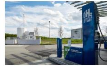
Stand-alone dispenser (e.g. for 700 bar and/or 350 bar)
