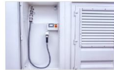
Integrated dispenser (e.g. 700 bar for mobile)
