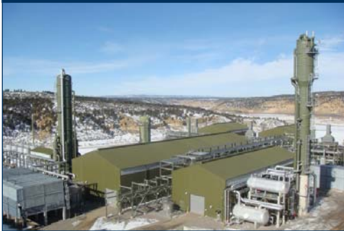
Natural gas processing plant
